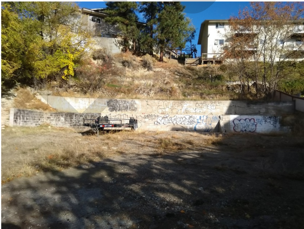
Figure 7: Rear Yard of Subject Property
